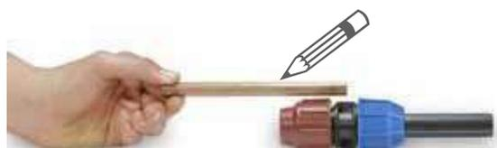
Chamfer the copper pipe end. Mark the pipe portion to be inserted into the fitting.
